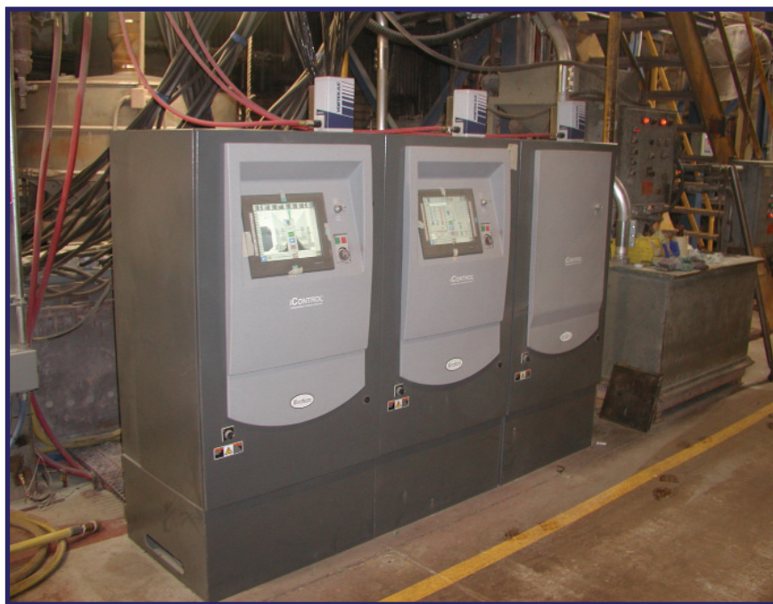
The compact size of the Vortex A/C units proved to be an important advantage when EB Pipe Coating purchased a new system that required three control panels to get 48 powder coating guns. The panels needed to be pushed up next to each other, which couldn't be done with conventional air conditioners mounted on the side of each panel
